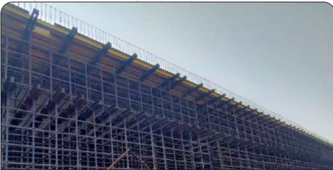
SAMRUDDHI MAHAMARG SITE
